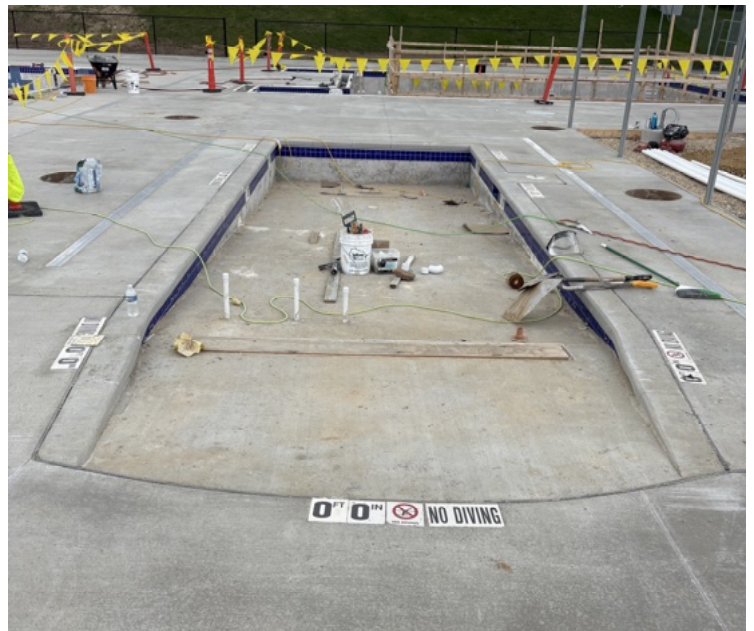
Pool tile install complete
