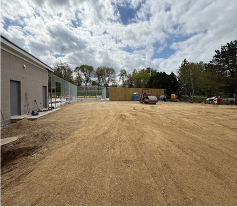
Tennis court graded and ready for paving
