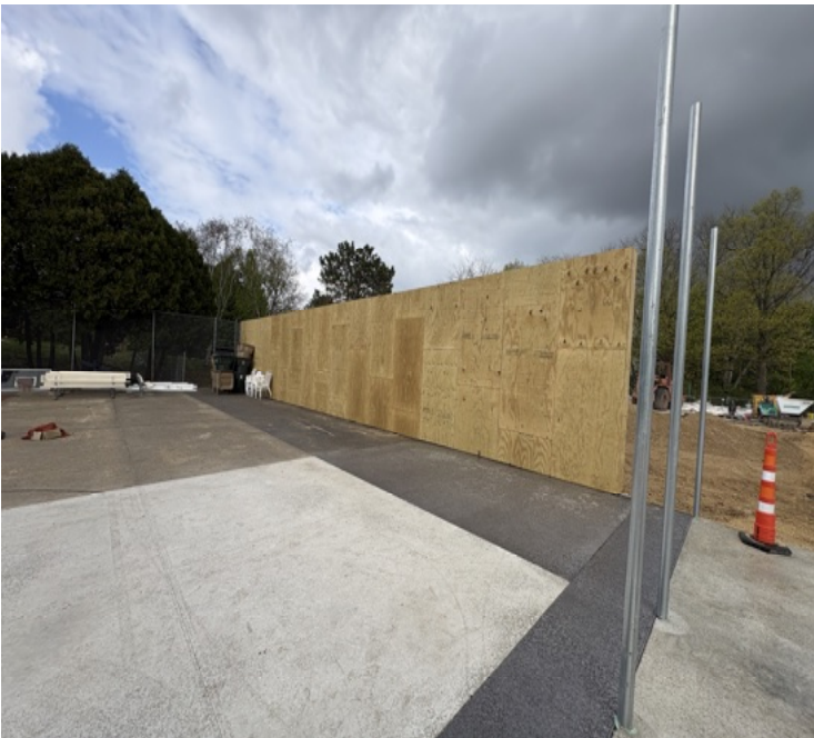
New wood wall installed
