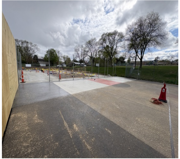
New basketball court colored concrete
