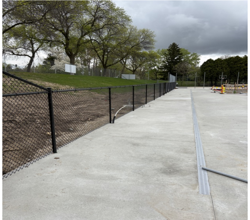
New fence, deck trench drains, and pool concrete deck
