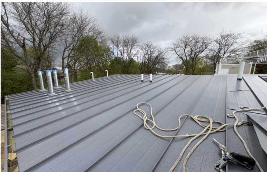
New roof and vent pipes installed
