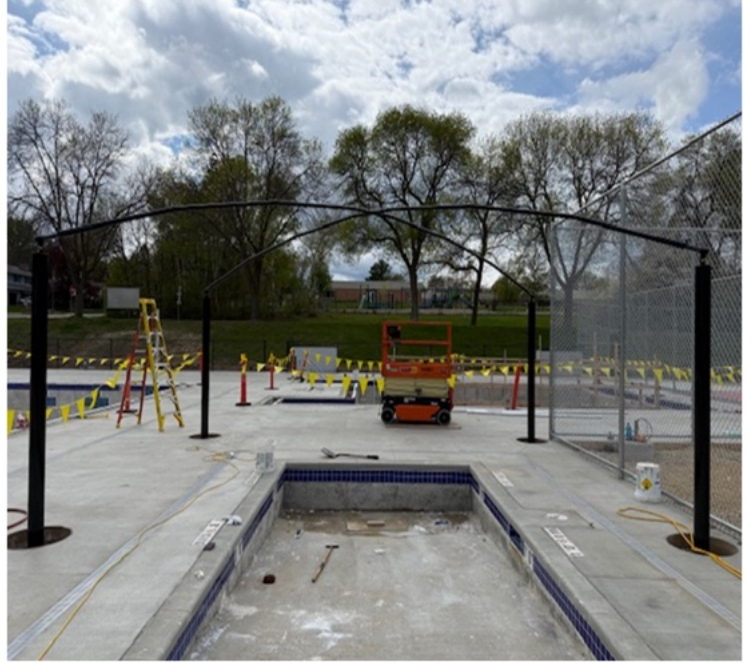
Shade structure installed
