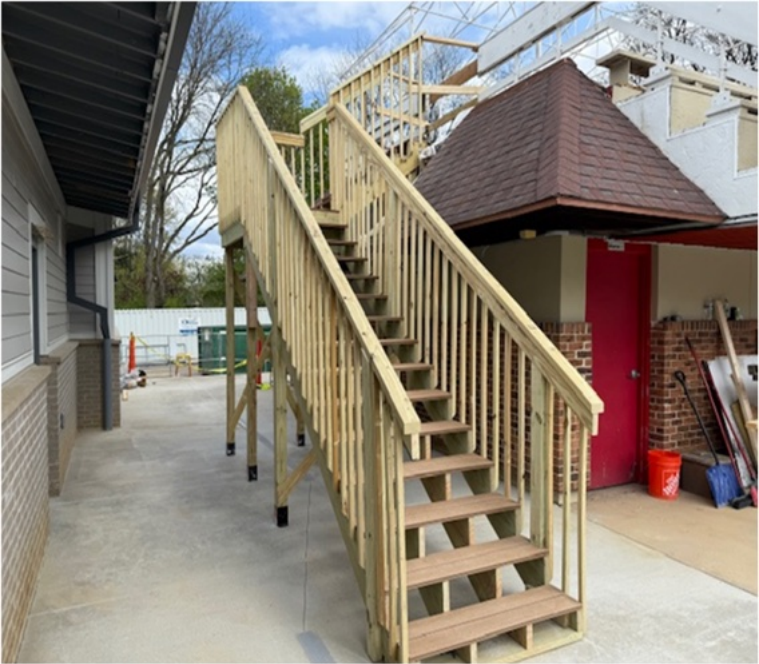
New wood pool house stairs
