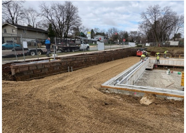
Retaining wall installed and backfilling for slab pour
