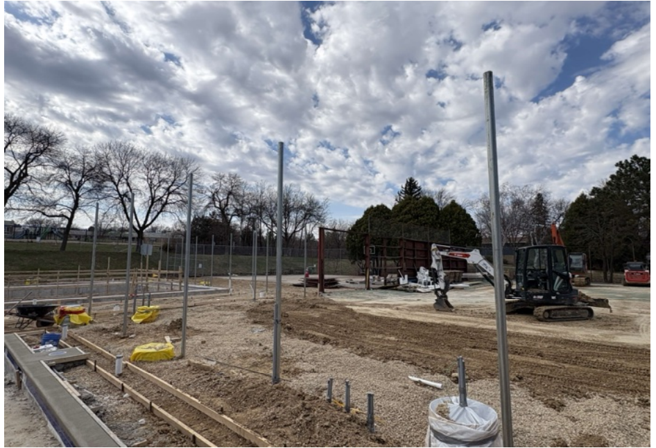
12-foot-tall fence posts installed
