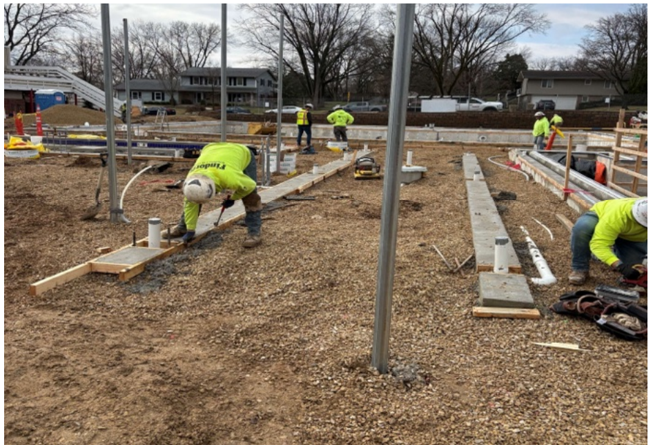
Deck trench drain footings poured out
