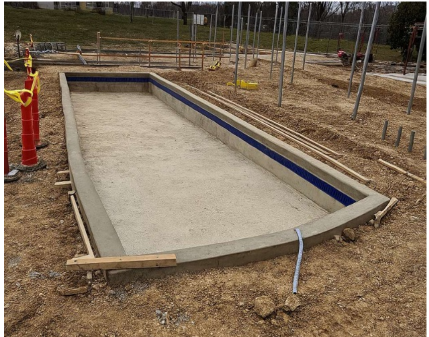
Wading pool progress
