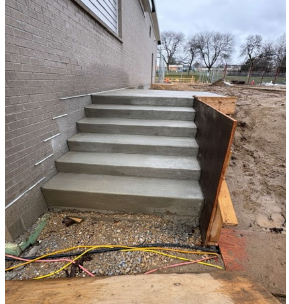
Exterior stairs poured out
