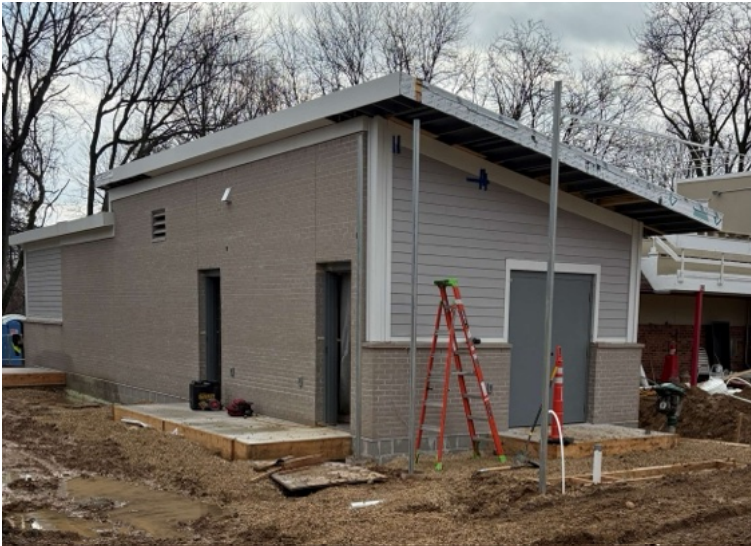
Cement board siding and door frames
