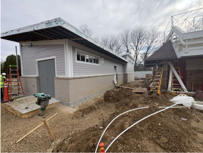
Mechanical building nearing façade finish
