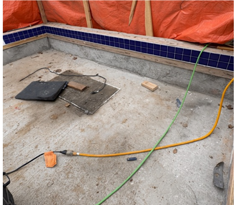
Tile installed within the wading pool
