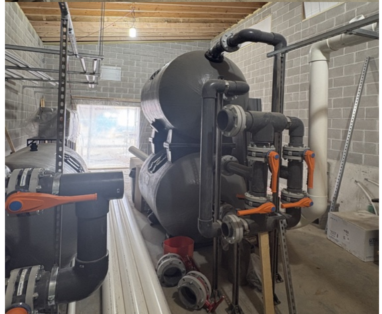
Pool Equipment Being Installed!
