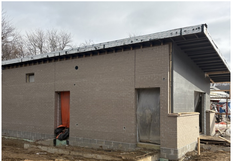
Brick Façade and Roof AVB Installed
