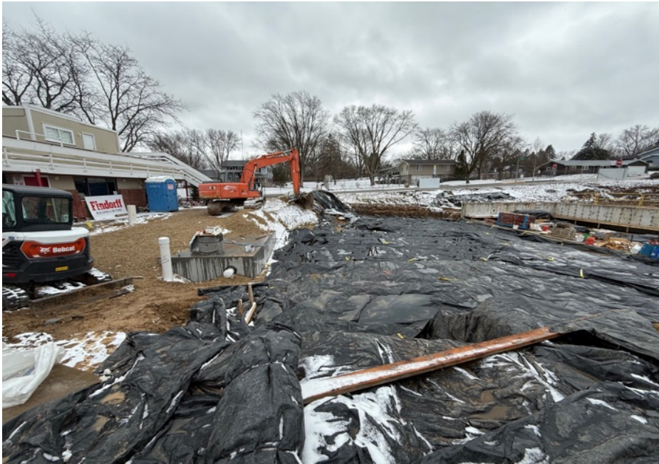
Excavation Work of Lap Pool Covered from the Cold
